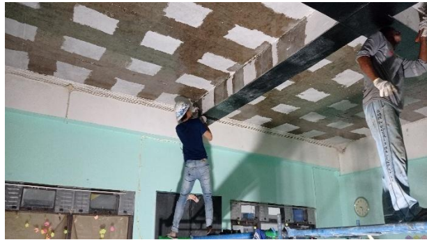
Figure 9. Utilizes epoxy resins or micro-cementitious grouts
