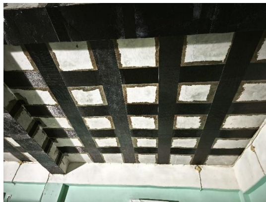
Figure 10. The application of Carbon Fiber Reinforced Polymer (CFRP)
