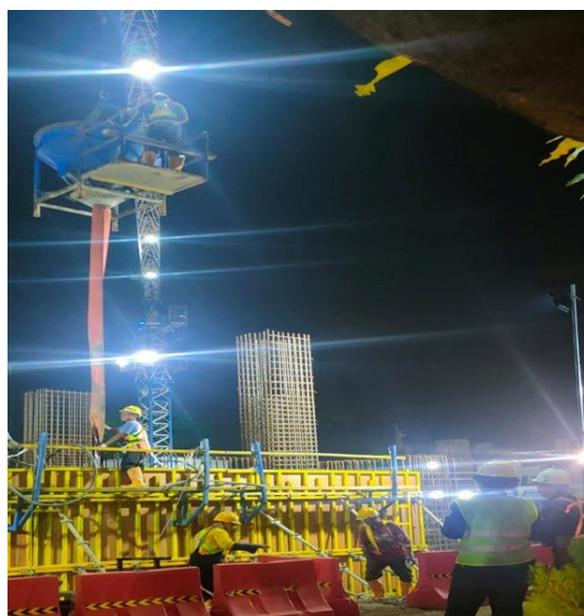
Gambar 8. Pengecoran Dinding Penahan Tanah
