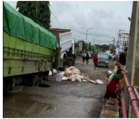
Figure 2. Subsidence that occurred in Oprit.
